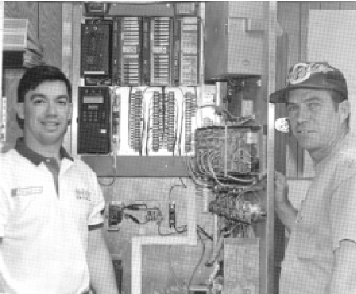
Chad Carpenter, left, of Tetragenics, and Bill Moritz, a city foreman in charge of the water system, stand in front of the new computerized control panel. Photo by Cindy L. Combs
